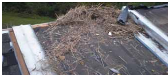
Figure 1. Cleaning the old shingle roof.
